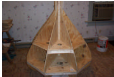
The beginning phase of the new cupola
